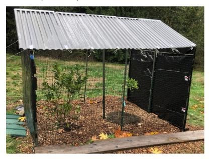
Here it is up close before the side panels were added, showing our two little friends. The roof is needed to handle a significant snowfall. Notice it's tied on with short pieces of rope. It's easy to remove, as are the end panels and the side panels roll down when the cold ends – or a windstorm is forecast. In summer, there's a relatively inconspicuous pipe skeleton that holds up the deer fence.
